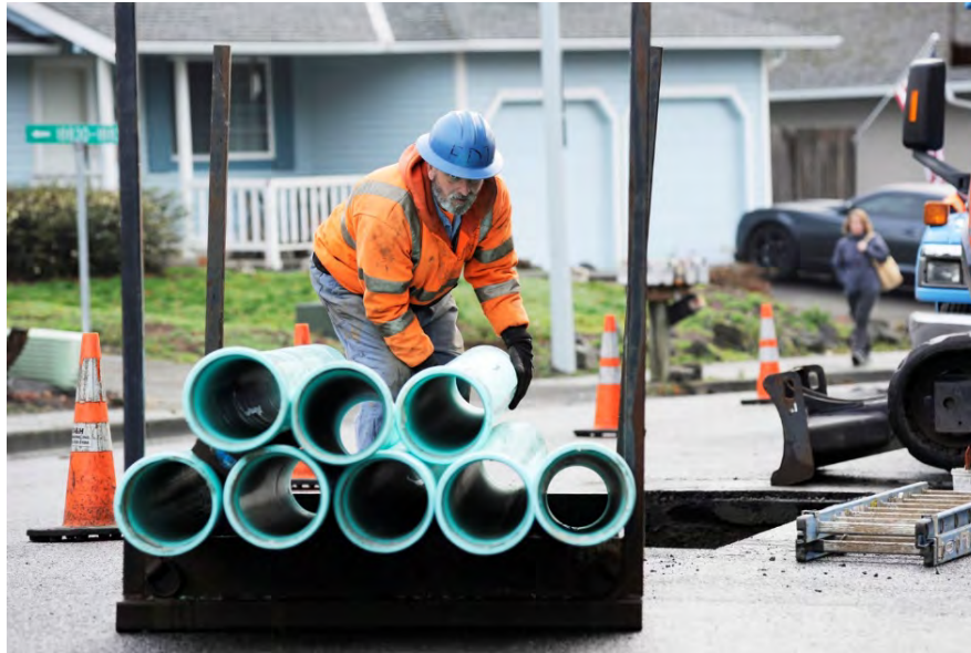
▲ Field Operations staff replacing section of collection system piping
