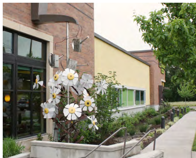
New Seasons, Beaverton. Two decorative scuppers collect and convey roof stormwater into an infiltration basin.
