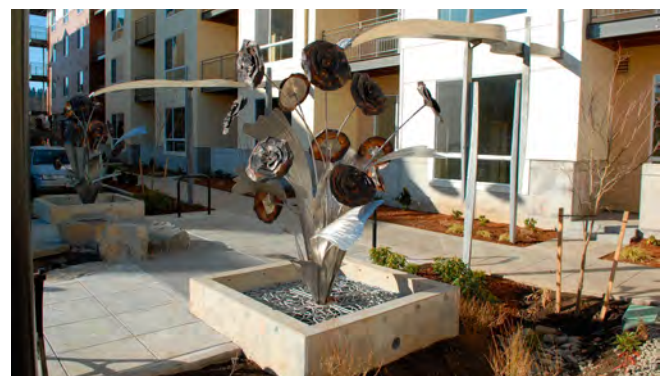
North Main Village, Milwaukee. Stormwater is the featured design element for this residential courtyard. Water from rooftops is conveyed by steel scuppers into decorative planters to meandering runnels and water quality swales.
