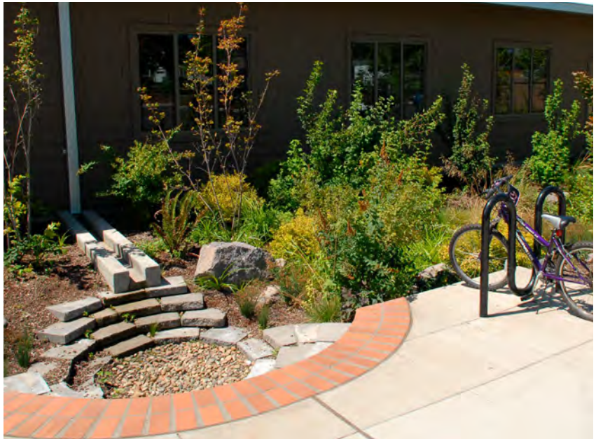
Estacada Library. Stormwater is conveyed from the rooftop to an infiltration basin. As the basin fills with water, it overflows into a connected series of swales and additional infiltration basins that convey stormwater around the library.
