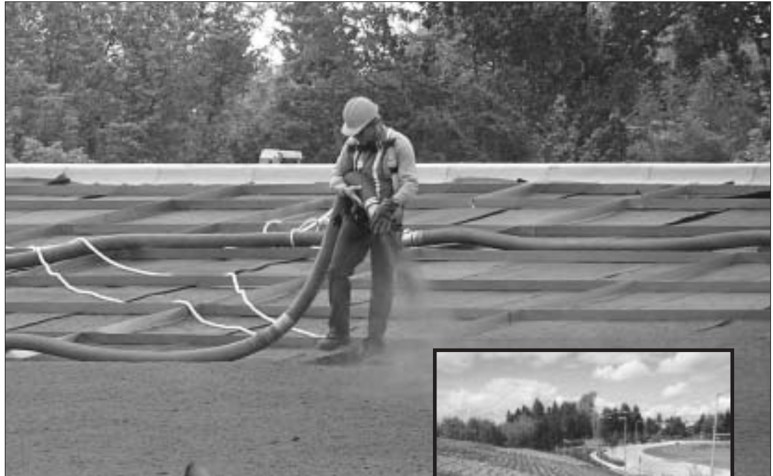
Blowing soil on the ecoroof
